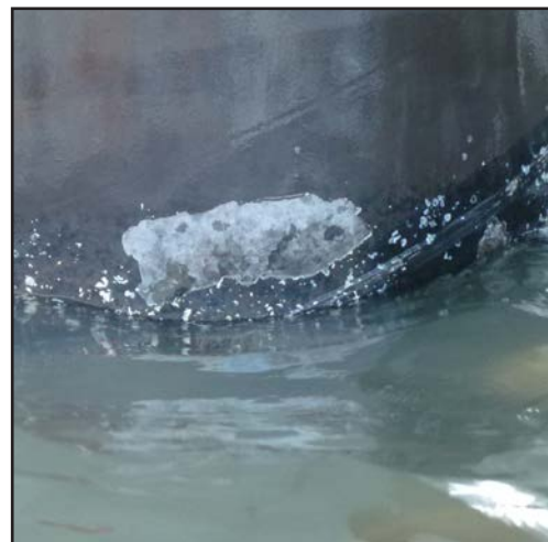
Example image of a pile featuring acceptable levels of non-living, tightly adhering mineral deposits.
