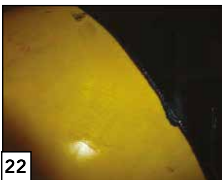
22 When sufficient temperature is reached, the texture on the sleeve will become smooth. The shrinking procedure is finished when the sleeve is tightly fitting everywhere and appears smooth.
