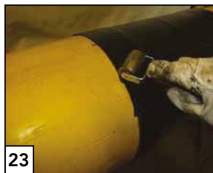
23 Roller the transition to the factory coating, the edge of the sleeve, the overlap of the sleeve and the area of the welded seam.
