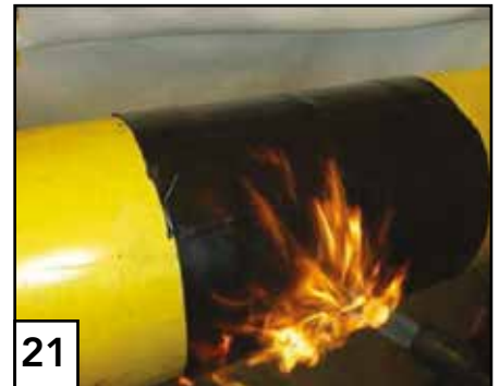
21 Beginning below, heat the middle of the sleeve, moving the torch in a circumferential direction with blue-yellow flame. Use the same motion to shrink one side, then the other side. Ensure even shrinkage.
