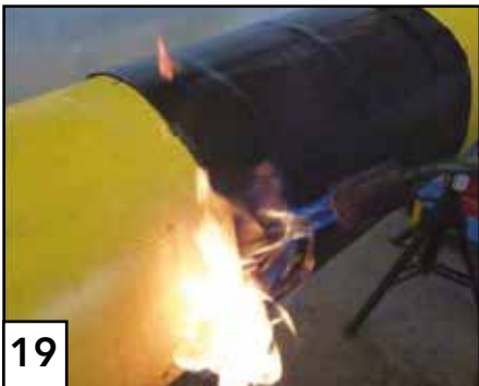
19 Continue warming the adhesive side of the closure patch and position it over the whole sleeve width in the overlapping area.
