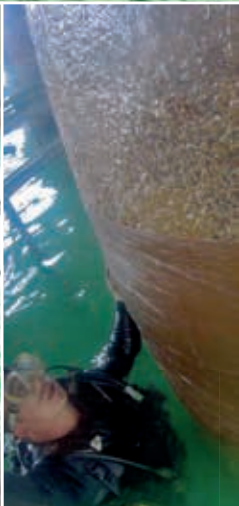
High pressure water jetting is used to prepare the surface before system application.
