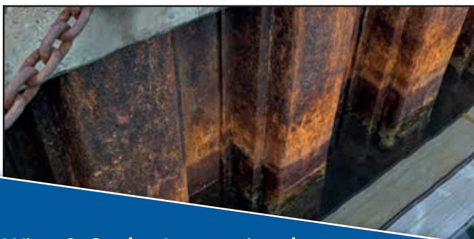
Below: Sheet pile wall before the SeaShield application.
