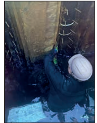
Application of Marine Piling Tape.
